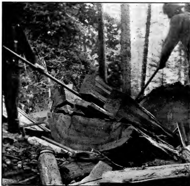
SPLITTING OUT THE TIES
